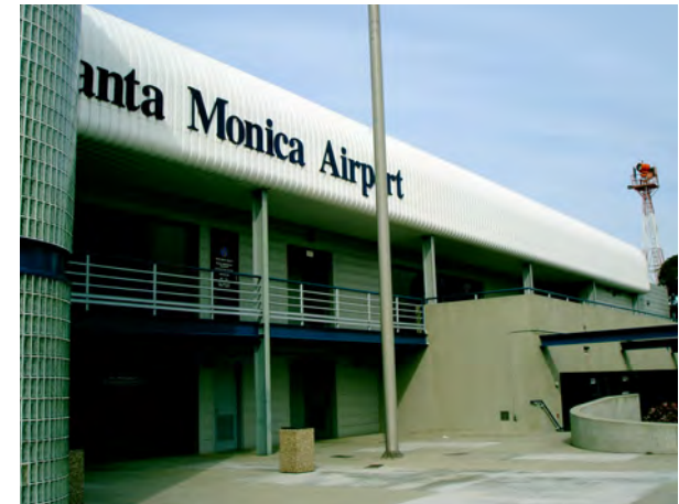
The “1984 Agreement” between Santa Monica and the federal government expires in 2015. The LUCE recommends a specific plan to explore the redevelopment of both the airport and the business park.
