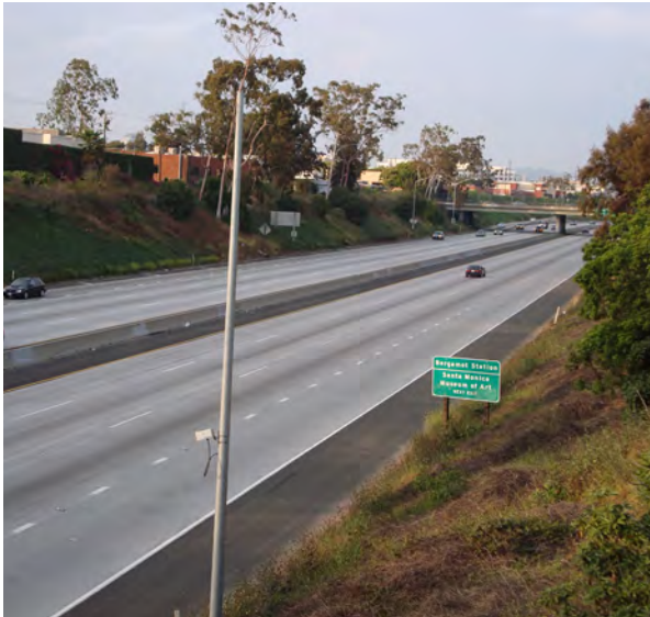
The construction of the I-10 Freeway created a permanent division between the north and south sides of the city.
