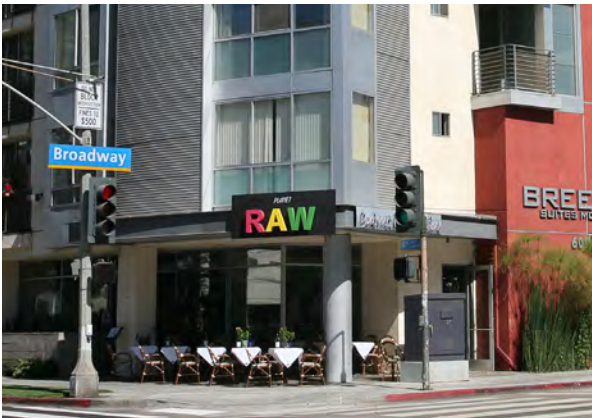
Active ground floor uses contribute to Downtown's livability, energy and completeness.
