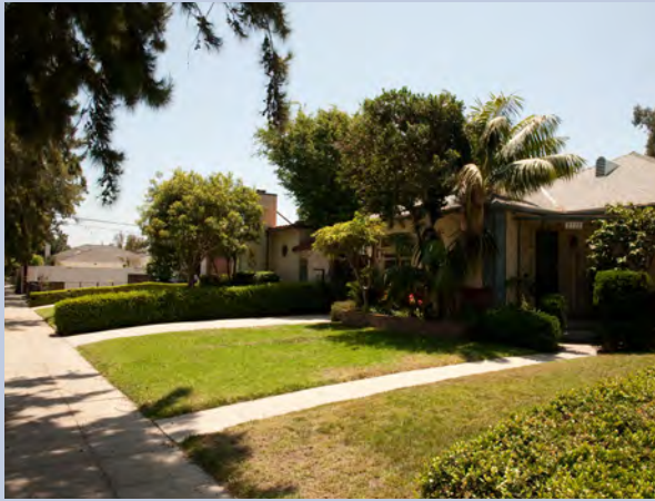
Conserving and protecting the quality and character of Sunset Park's single and multi-family housing stock is a primary objective of the LUCE.
