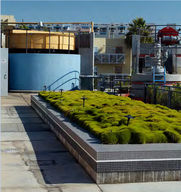
Water quality is a major resource issue, and one that Santa Monica takes very seriously. The SMURRF, pictured above, treats dry weather urban runoff before it enters the Bay.
