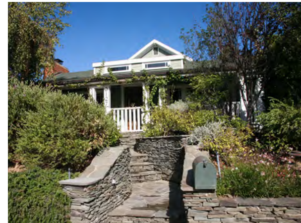
The smaller single family homes of Sunset Park reflect the area's history as a working class residential neighborhood.
