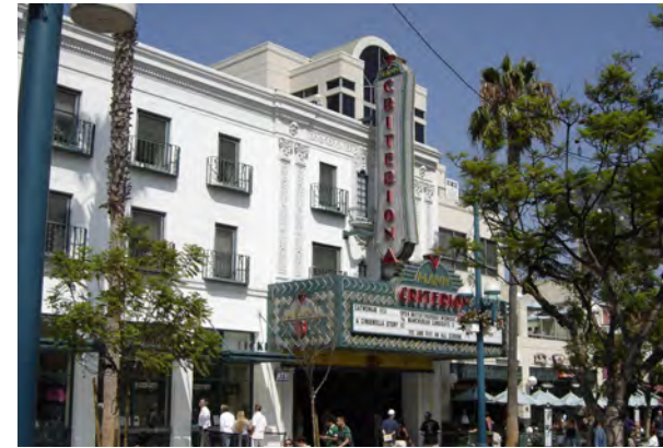
Downtown Santa Monica is home to many mixed-use buildings, including the historic Criterion Building constructed in 1924.
