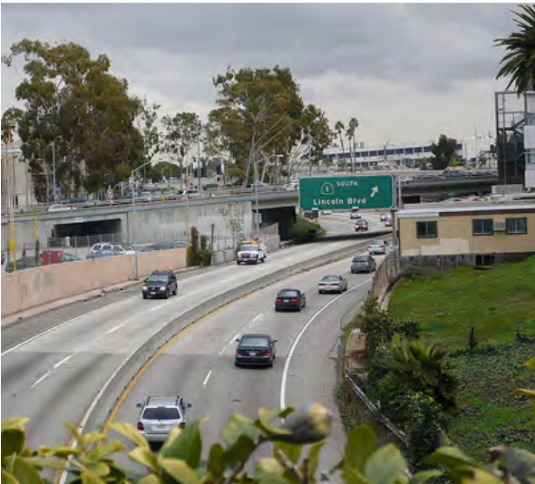
Cleaner air: Under the LUCE, some new development projects will pay into a fund to mitigate the pollution created from trips the projects create.
